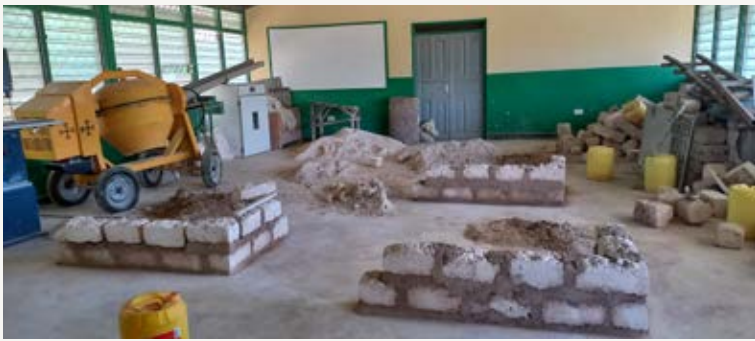
◀ Masonry workshop at Likoni Rehabilitation School.
